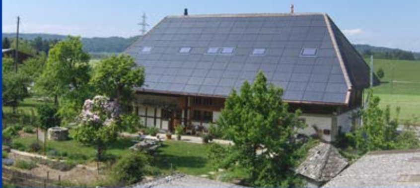
Fam. Wüthrich, Uettligen/BE (1819): 23 kWp - 22'500 kWh/a
